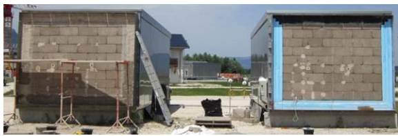
Figure 1 : Passys cells with hempcrete walls
